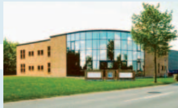
The Partner Voxstream premises in Vamdrup, Denmark
