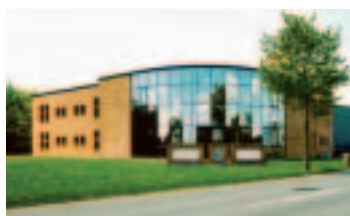
The Partner Voxstream premises in Vamdrup, Denmark
